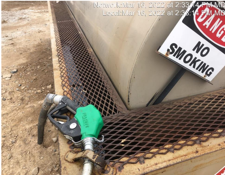
Photo #6204 . Insufficient maintenance of material handling and spill prevention BMP's. Containment full of an unknown fluid.
