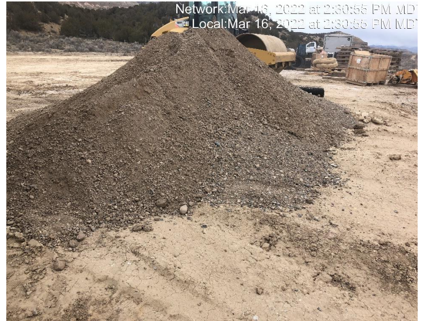
Photo #6202 Insufficient materials covering and BMP implementation.
