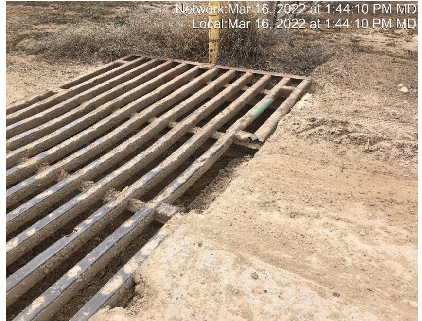
Photo #6199 Insufficient tracking BMP at entrance to location.
