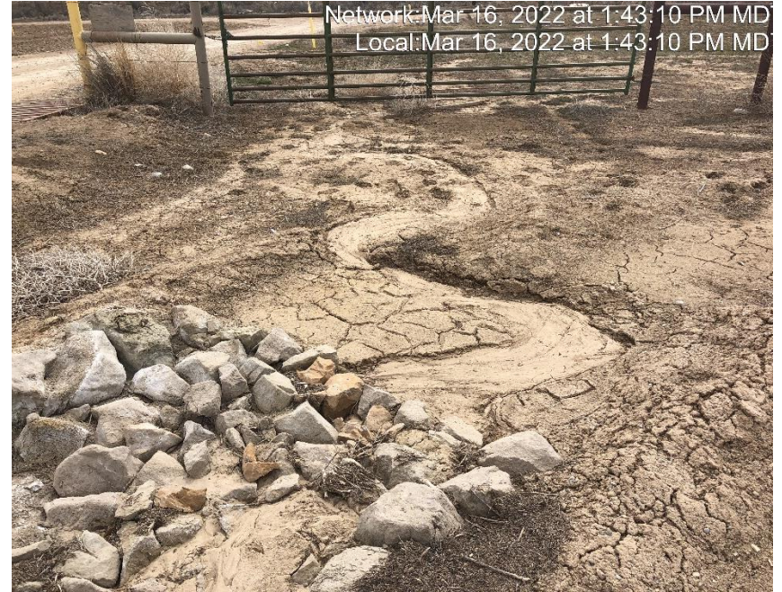
Photo #6196 sediment trap insufficient.
