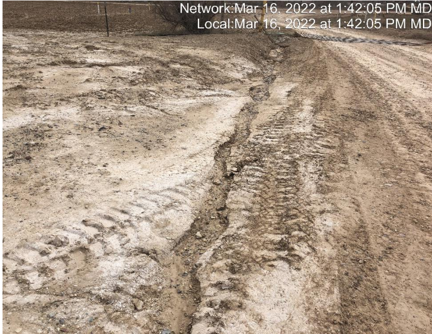
Photo #6193 Rill erosion occurring on location.
