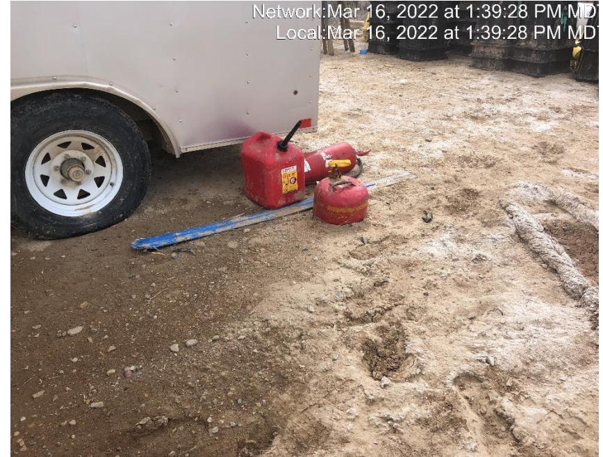
Photo #6188 Material handling and spill prevention BMP's have not been implemented.
