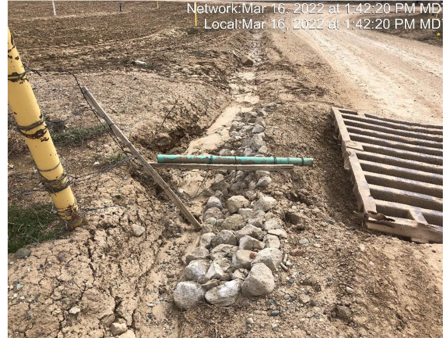
Photo #6194 Sediment trap insufficient.
