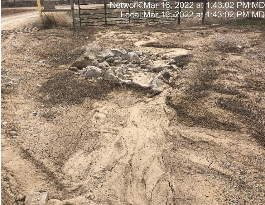
Photo #6195 Sediment trap insufficient.
