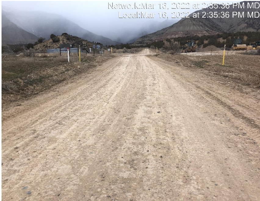
Photo #6205 Insufficient tracking BMP at entrance to location.
