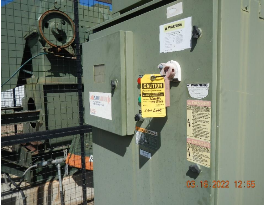
The pump controller for C #2 is tagged out.
