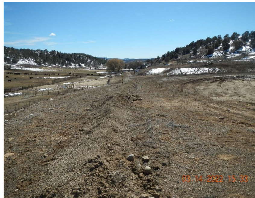
Recently installed perimeter berm.
