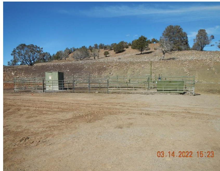
"Pump to line" system (right side of photo) has recently taken the place of the vertical heated separator.
