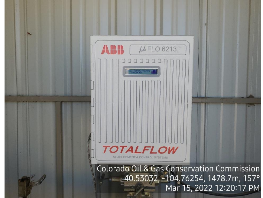
Photo 6: No calibration card displayed
