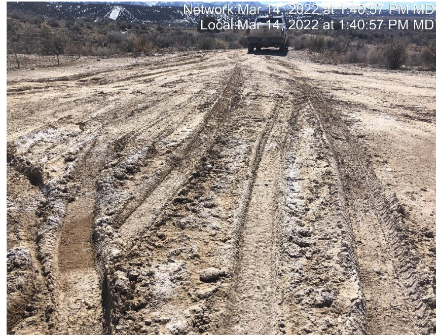
Photo #6164 Insufficient tracking BMP at entrance to location.
