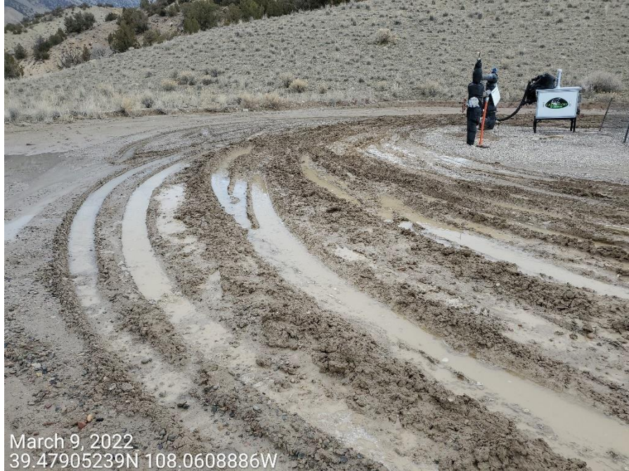
Photo 3: Photos taken from the working pad of the Location. Photos provide examples showing control measures to stabilize the working pad, minimize rutting, tracking and sediment transport remains missing or insufficient.
