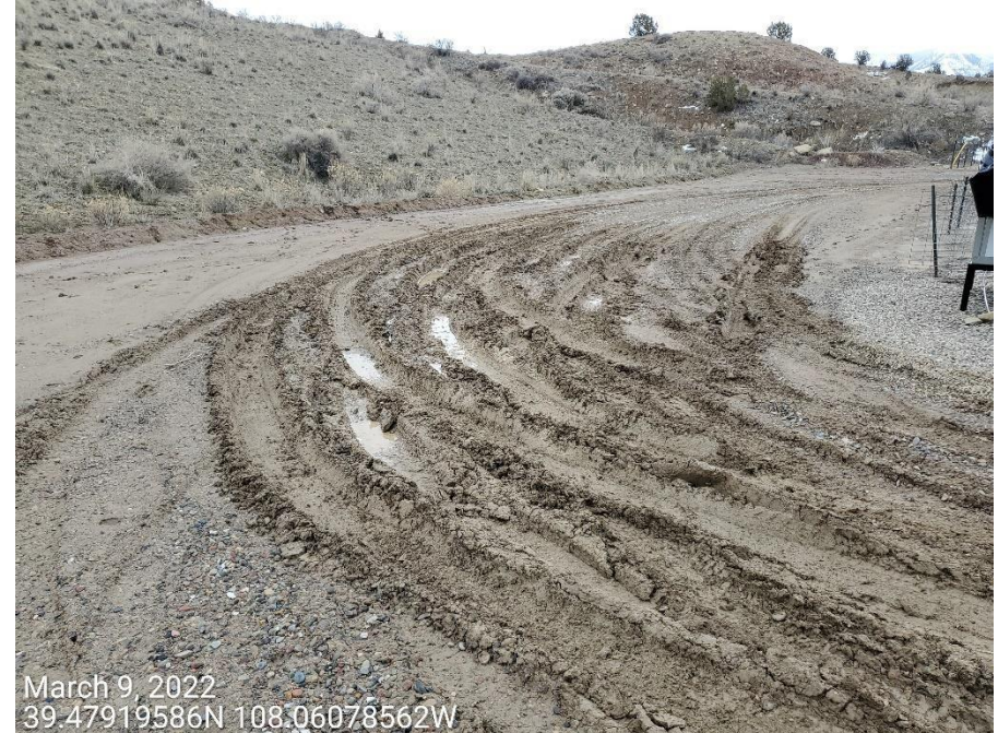
Photo 3: Photos taken from the working pad of the Location. Photos provide examples showing control measures to stabilize the working pad, minimize rutting, tracking and sediment transport remains missing or insufficient.
