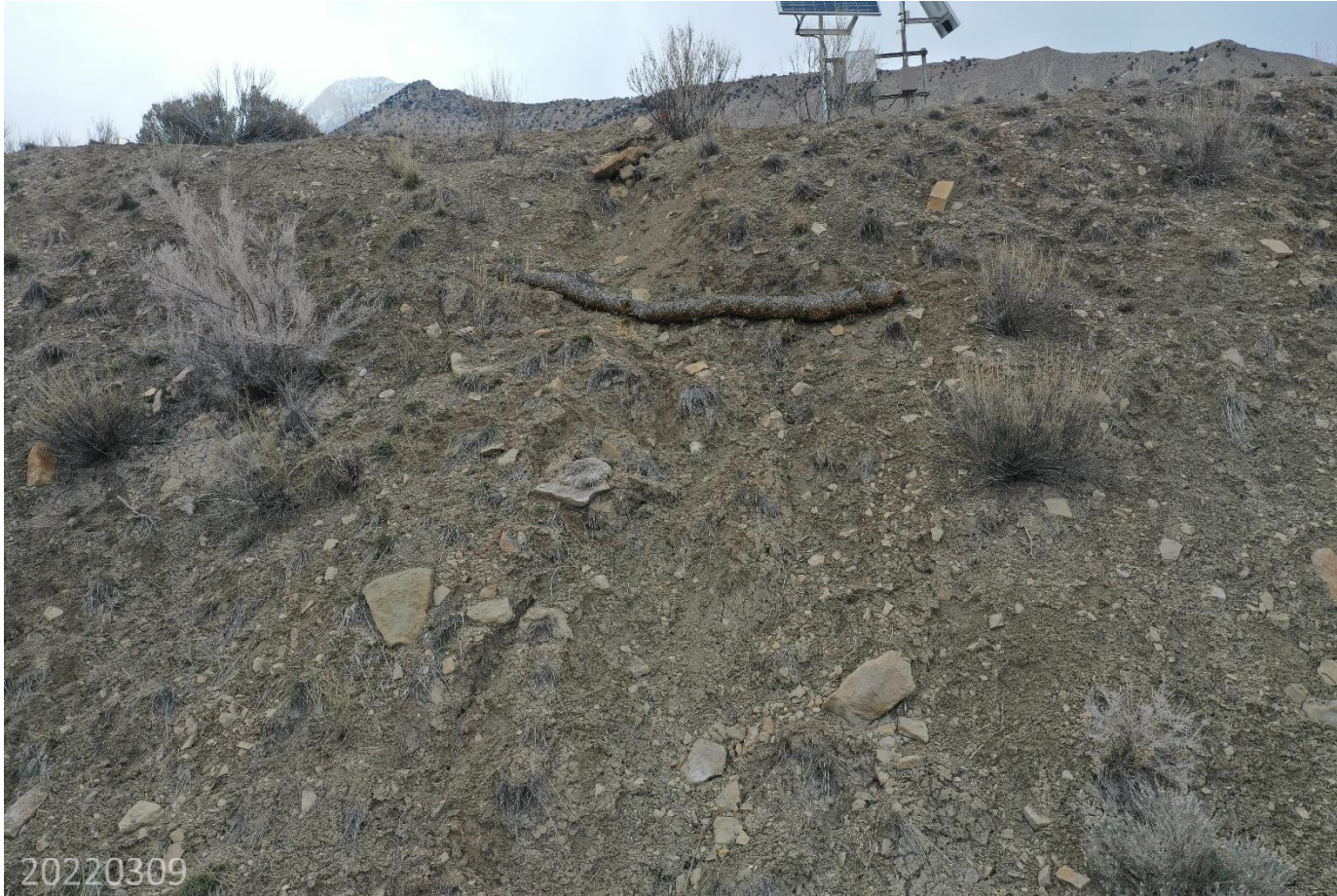
Photo 8: Photo taken with use of a sUAS. Photo taken from northwest end of the Location, facing southeast. Photo provides an overview of the Location showing control measures to stabilize the working pad, minimize rutting, tracking and sediment transport remains missing or insufficient.
