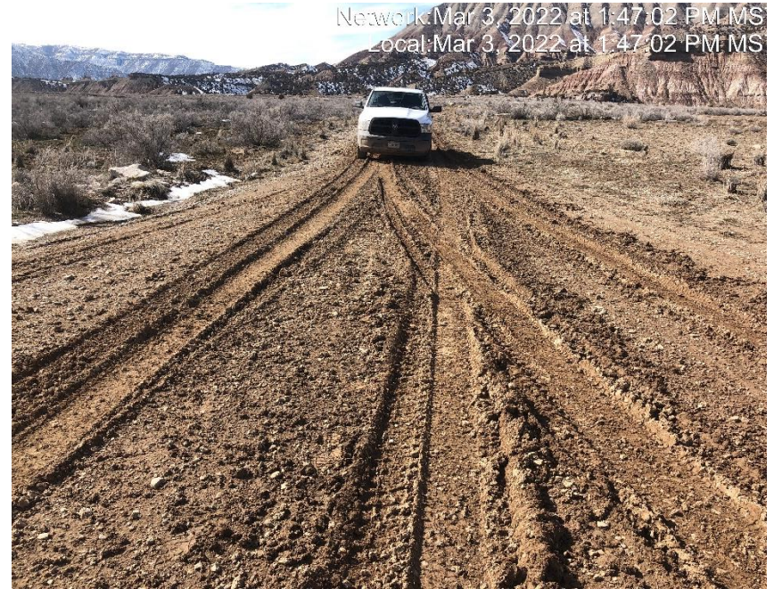
Photo #6083 Insufficient tracking BMP at entrance to location .
