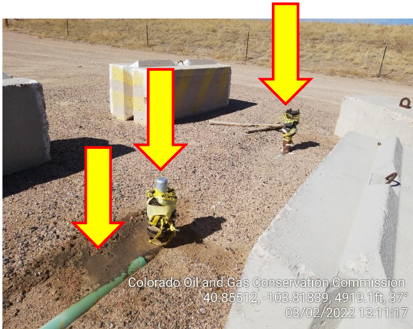
Photo 3 – Unmarked Risers and Stained Soil West of Compressors
