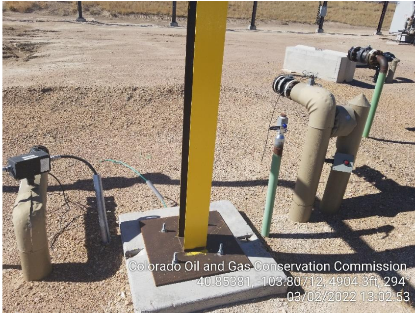
Photo 9 – Unmarked Risers
