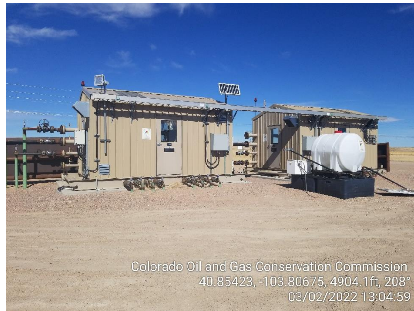
Photo 14 – Gas Lift Injection Meter Sheds
