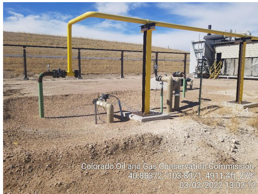
Photo 8 – Unmarked Risers
