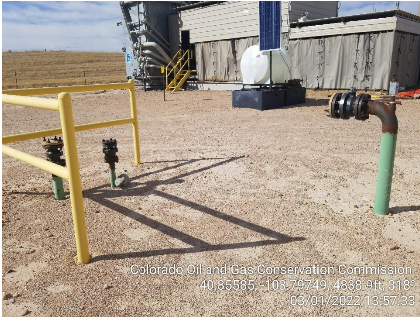
Photo 17 – Unmarked Risers
