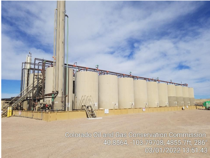
Photo 5 – Tank Battery
