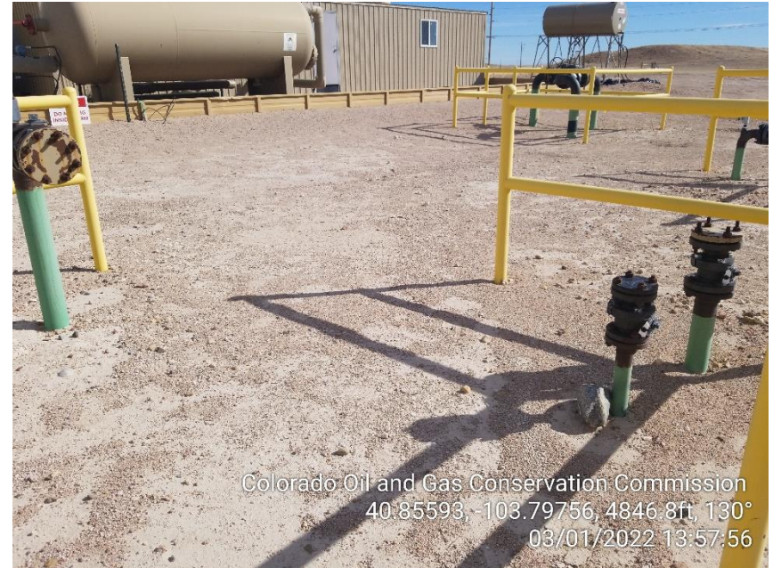
Photo 18 – Unmarked Risers
