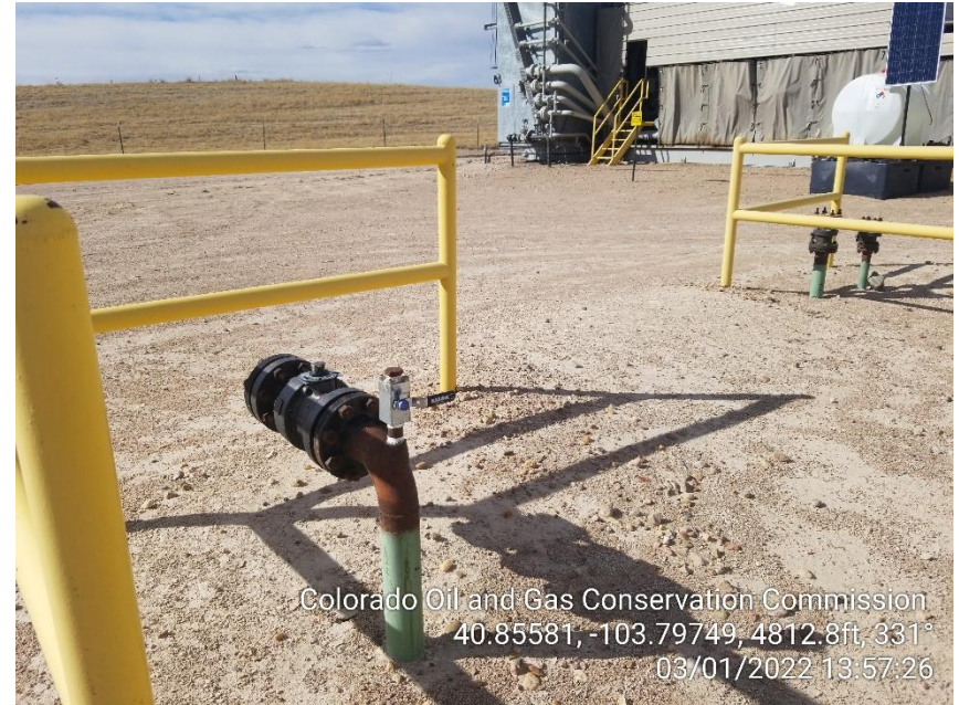
Photo 16 – Unmarked Riser
