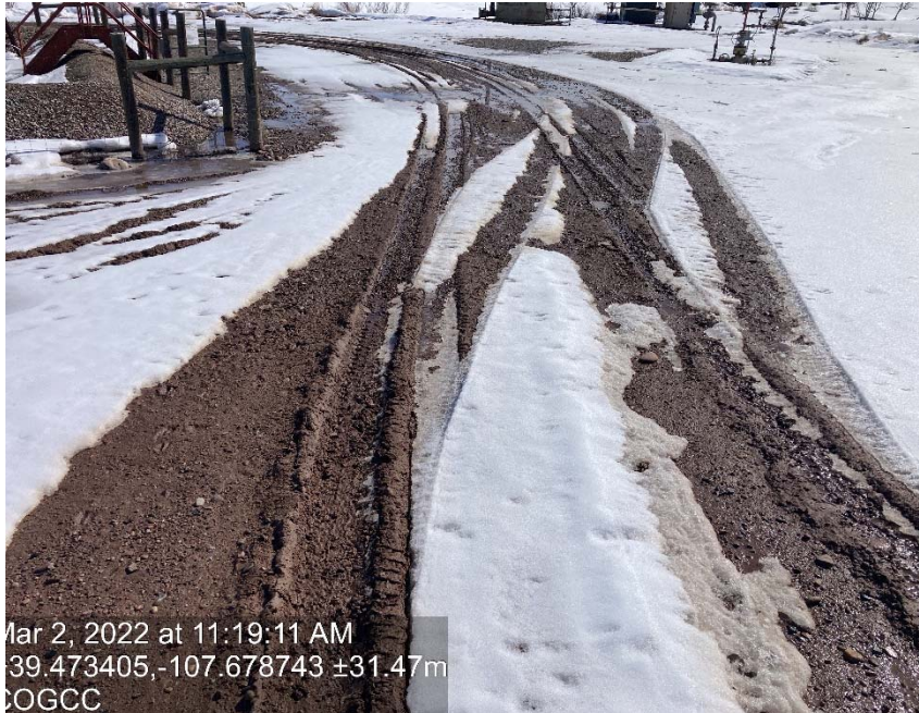
Lack of stabilization/compaction
