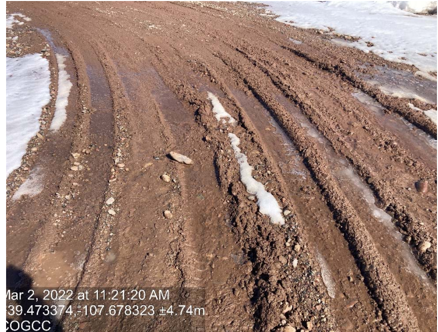
Lack of stabilization/compaction
