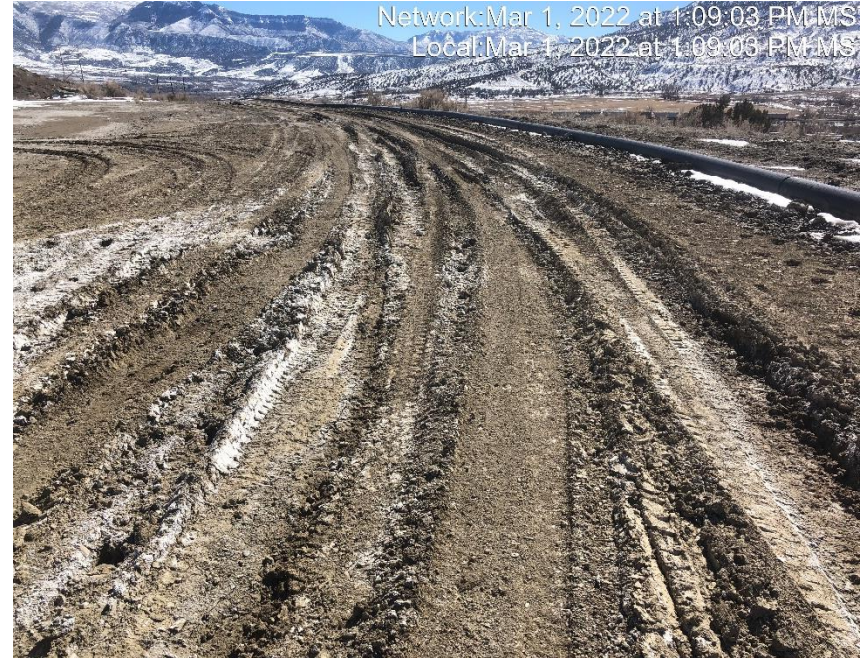
Photo #6060 Insufficient tracking BMP located at entrance to location.
