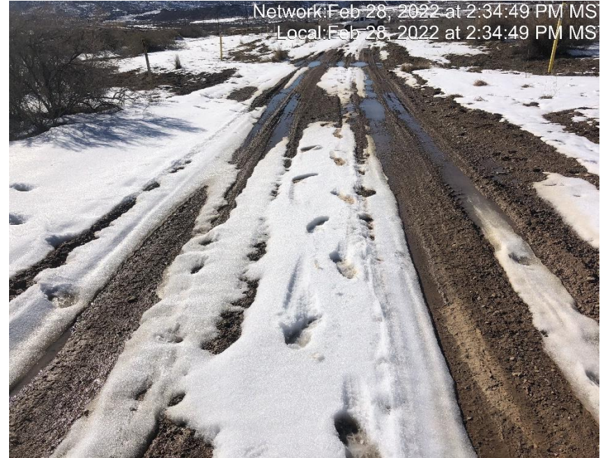
Photo #6055 Insufficient tracking control at entrance to location.
