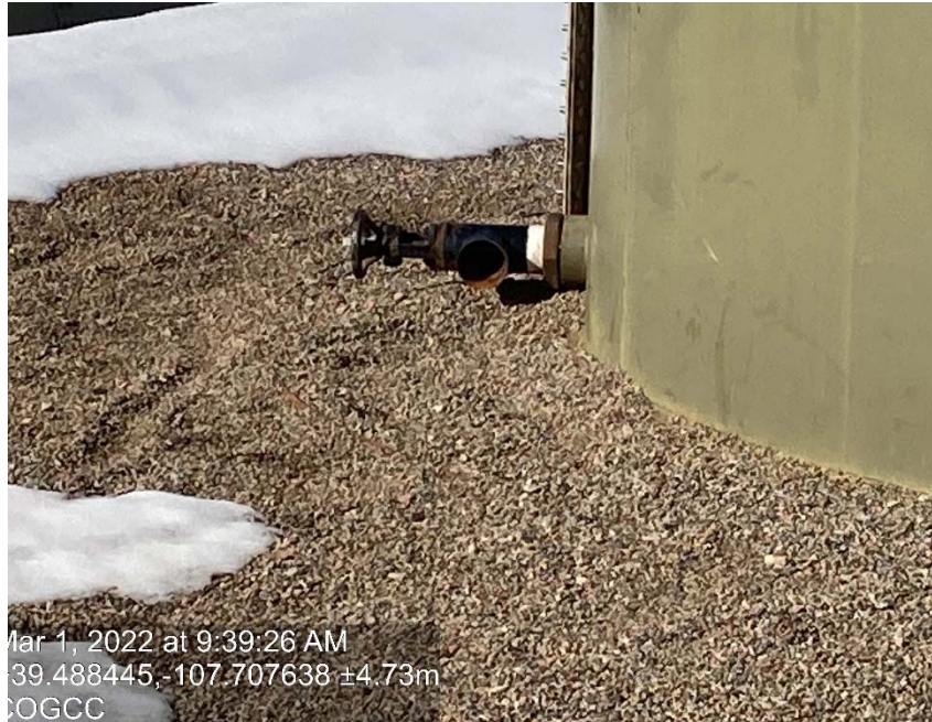
Line missing plug/cap
