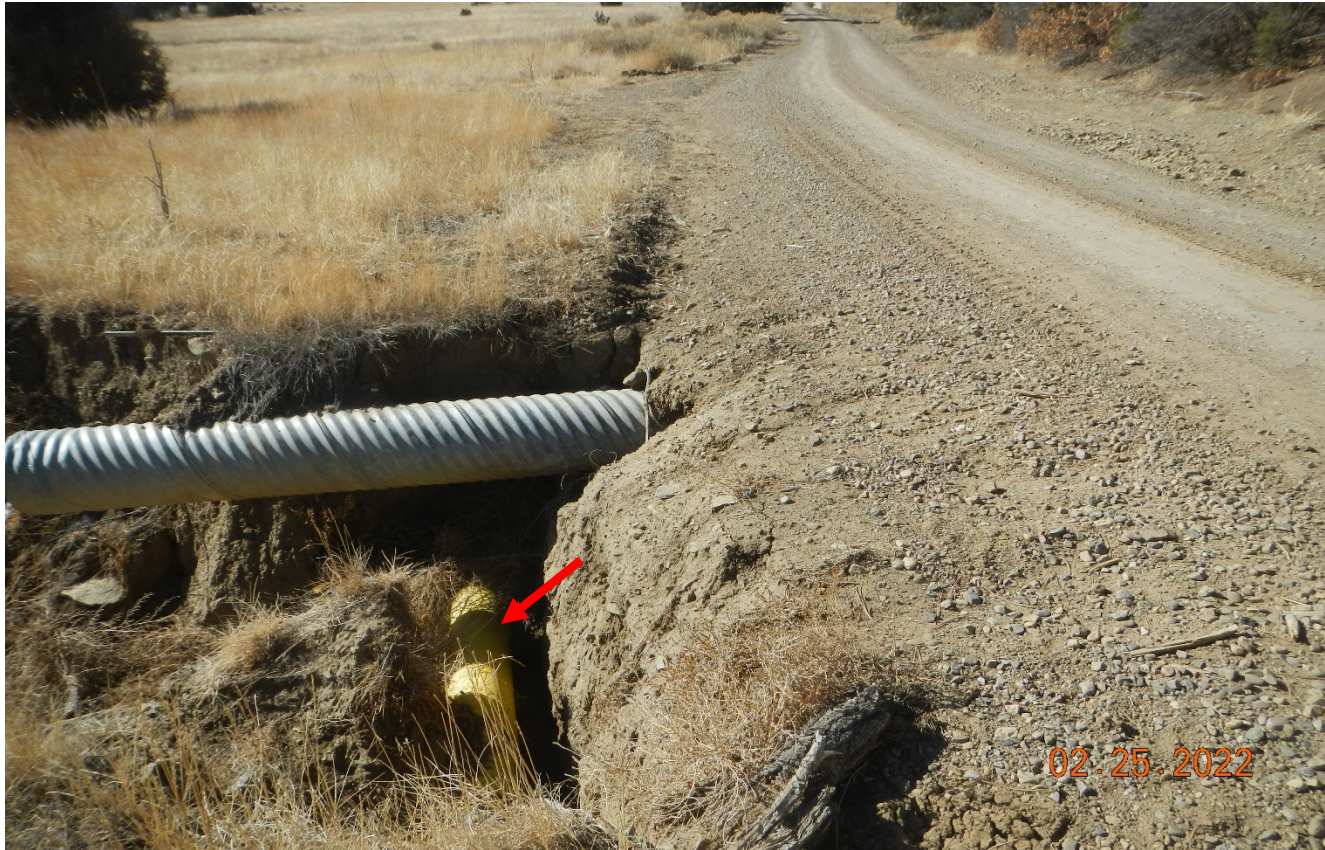
Photo 3. This culvert along the main road is partially washed out and needs to be repaired. There is an exposed pipeline shown at red arrow.
