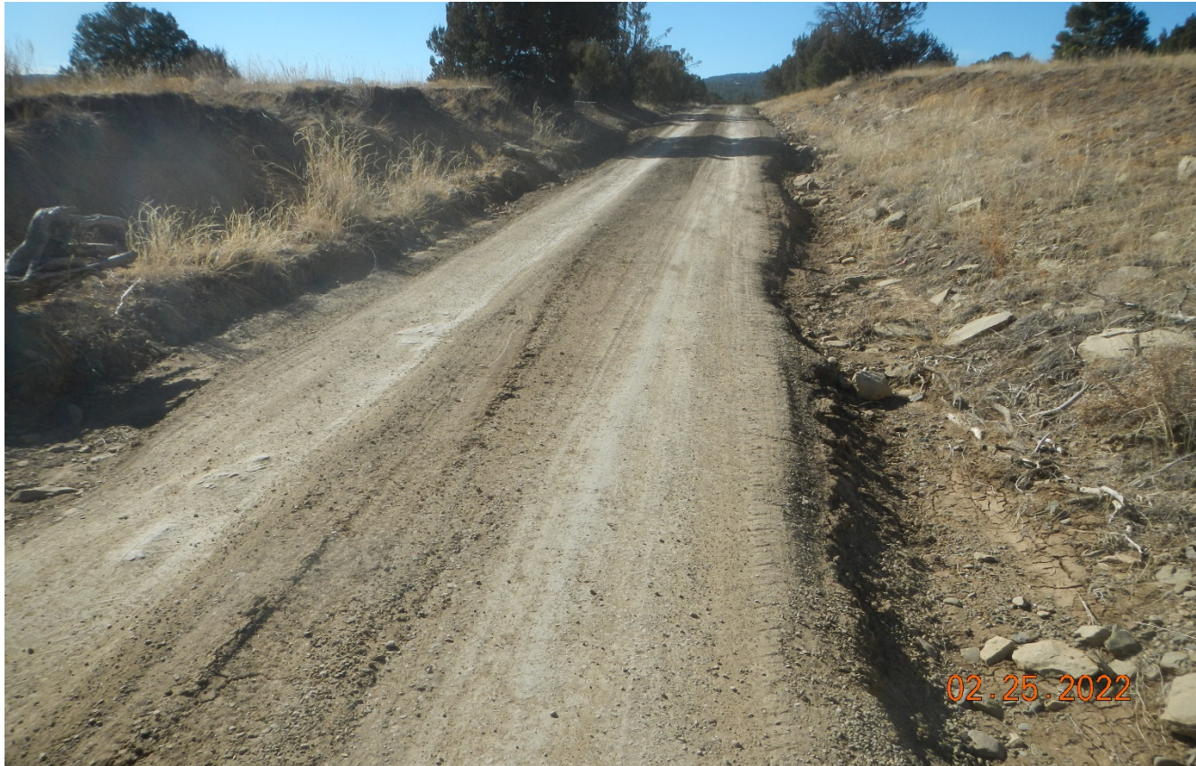
Photo 1. Facing southwest along the main road near the electric gate. Stormwater is directed down the road side in this area which is contributing to erosion further down the county road.
