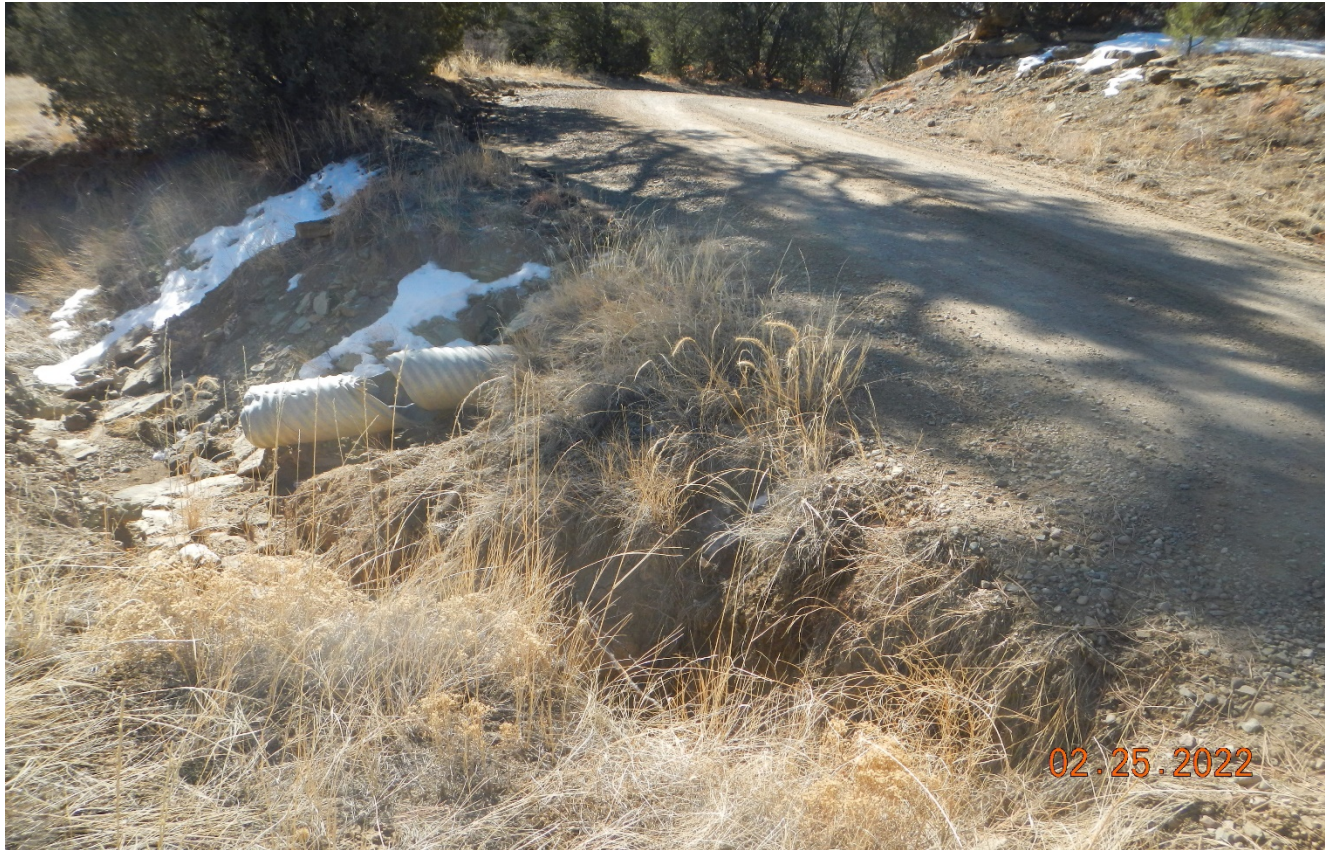
Photo 2. This culvert along the main road is partially washed out and needs to be repaired. Lat/Long:37.08136,-104.62910.
