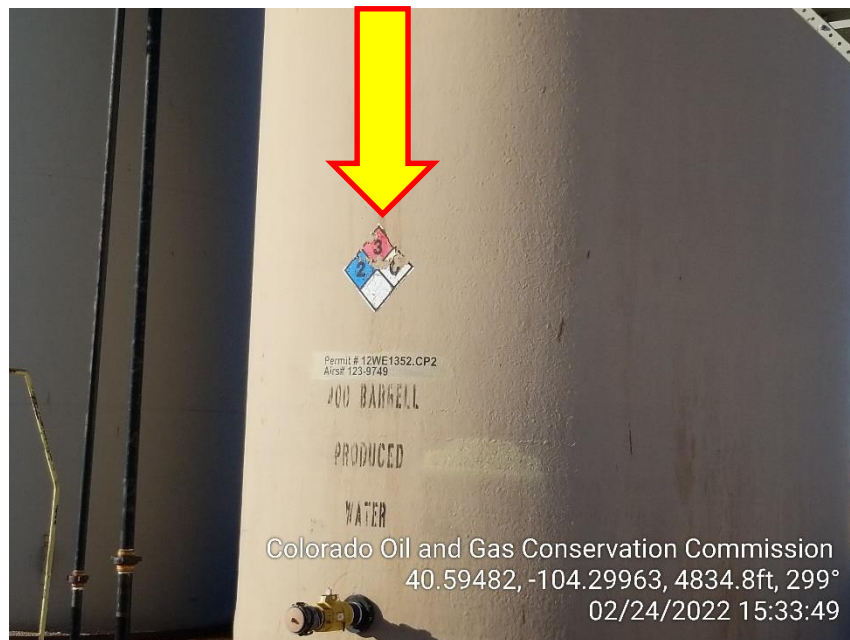
Photo 7 – Produced Water Tank NFA is starting to fade
