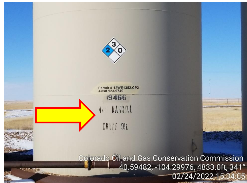
Photo 8 – Content and Capacity on Middle Oil Tank is starting to fade
