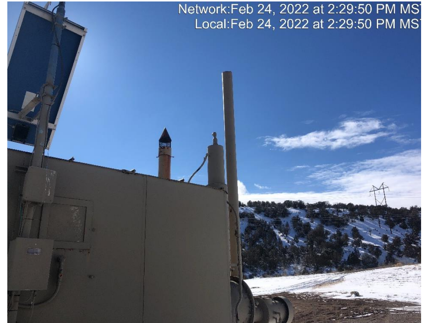
Photo #6026 Burner stack missing bird protector.
