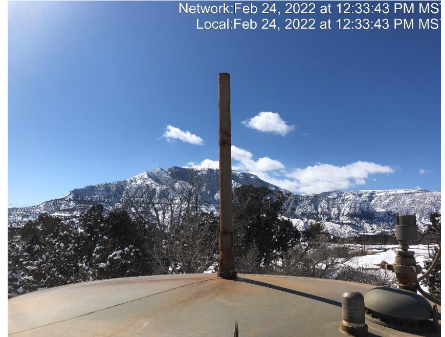
Photo #6012 Vent pipe on tank open ended.
