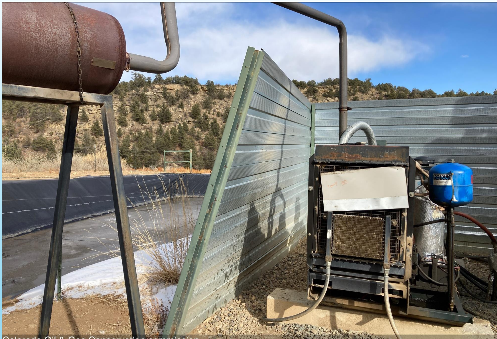
PHOTO 10: SOUND WALL IS LEANING AND WILL NEED REPAIR SOON.
