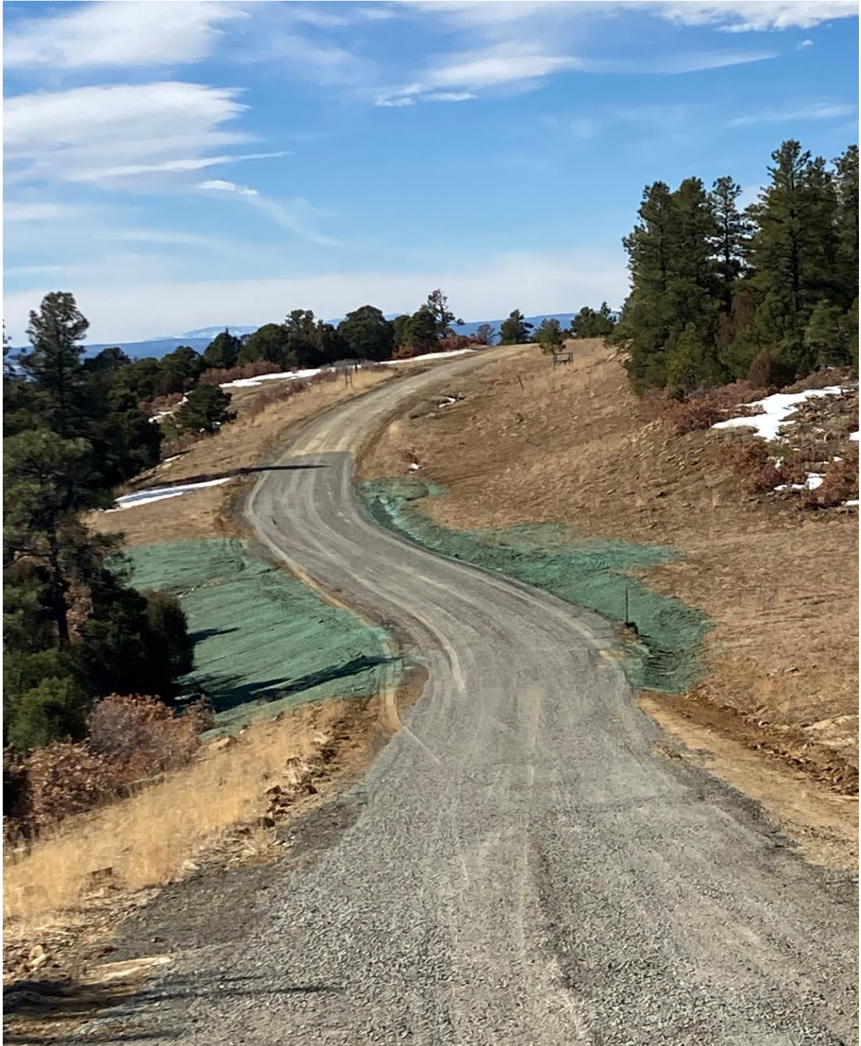
The road near the well site has been repaired. The erosion and the side of the side of the road has been stabilized. Stormwater was diverted toward the culvert. Areas of erosion repaired and stabilized. Repairing required BMPs per Rule 1002.f.(2)C.
