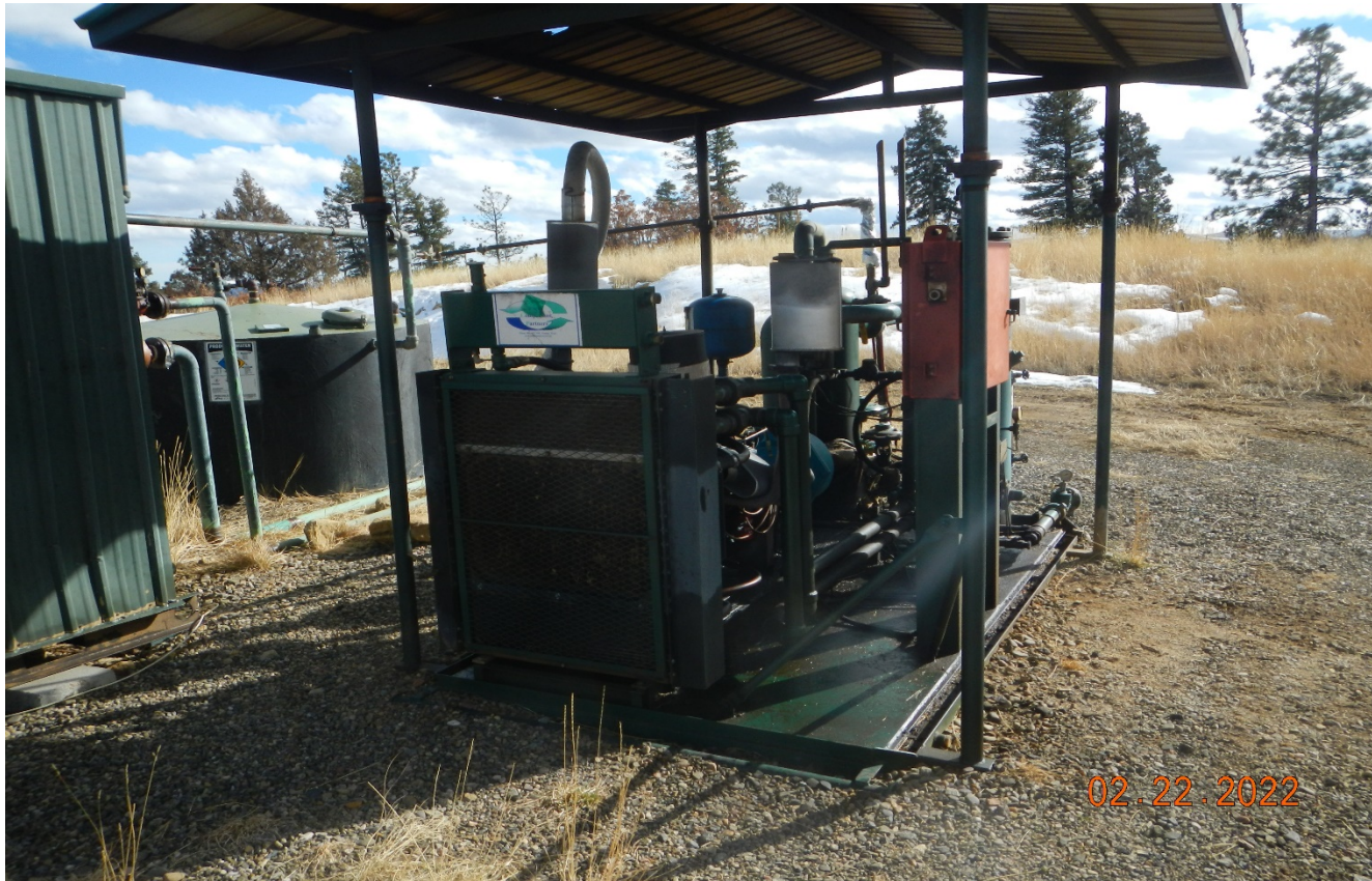
Photo 3. The engine is abnormally loud and it looks like the muffler needs maintenance.
