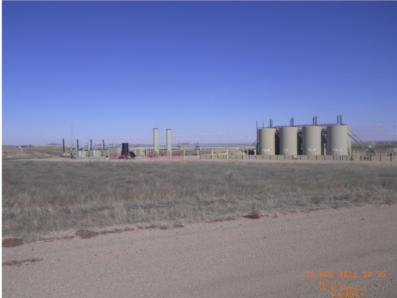
Photo 3. Tank battery remains for the producing wells on site.
