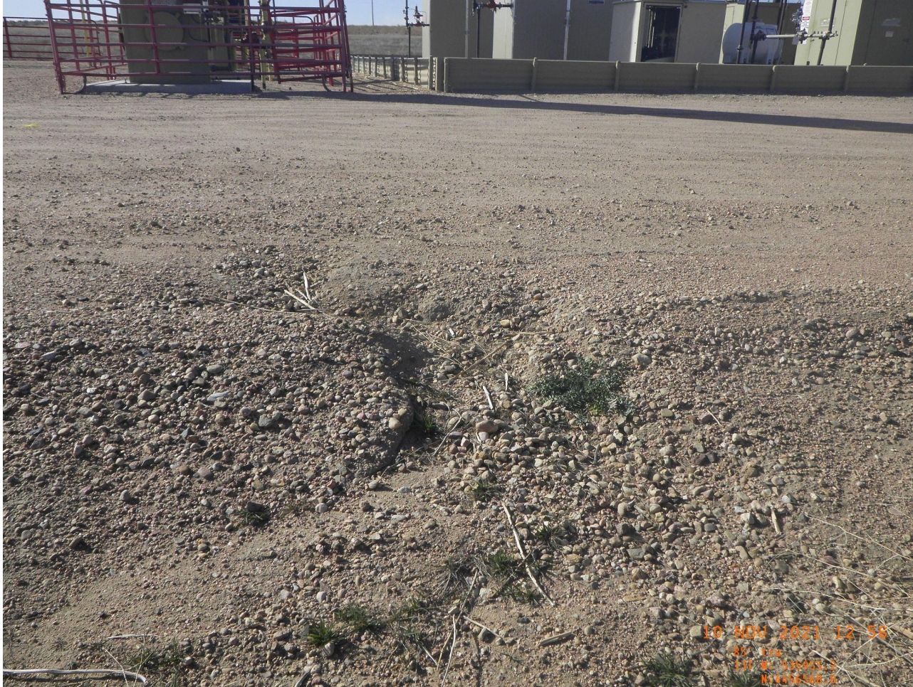
Photo 4. Rill erosion observed on the northeastern edge of the tank battery.
