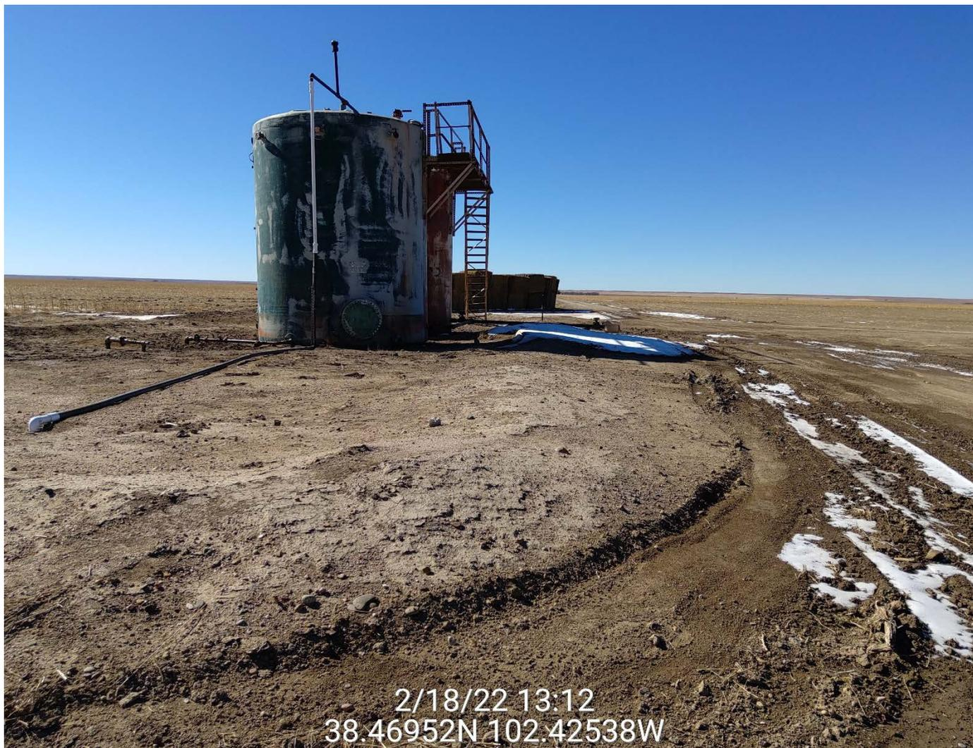
Containment around tank battery is inadequate
