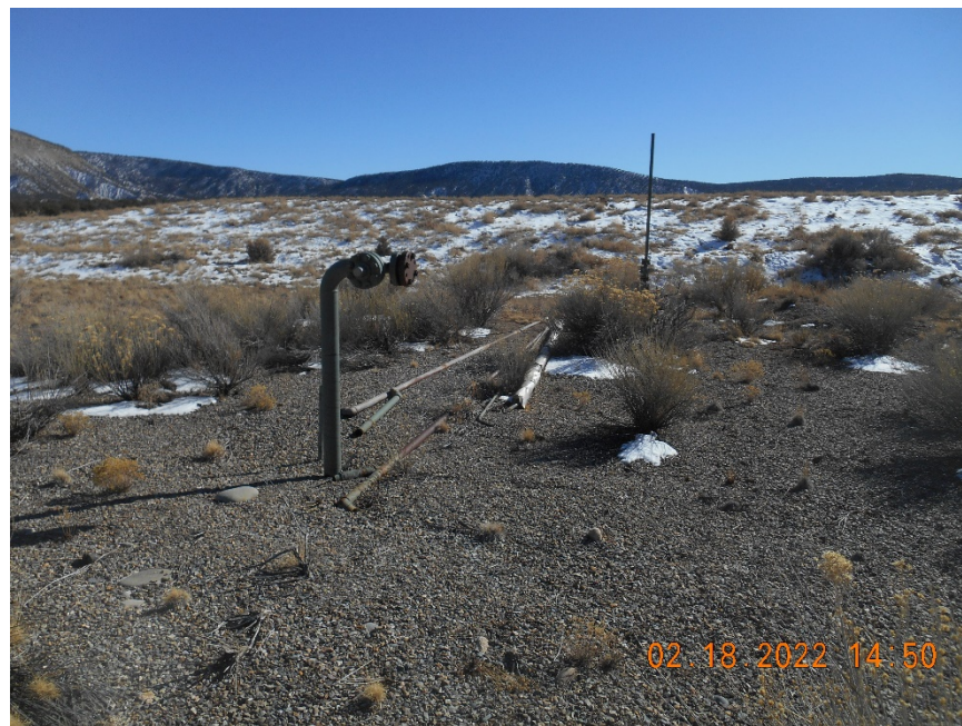
Flowline riser locked out/tagged out Unused flowlines
