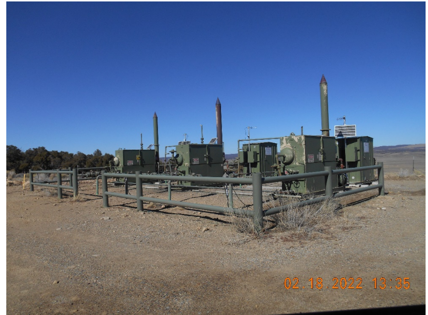
Separators and Meter housings
