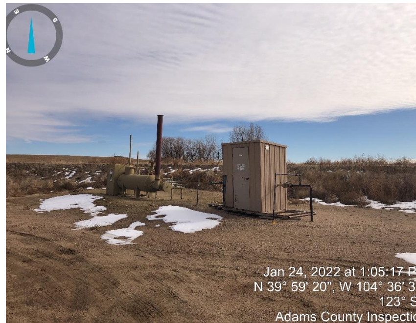
Photo #2 Meter & Separator.
