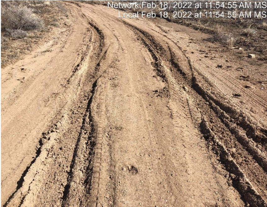
Photo #5992 Access road lacks stabilization.
