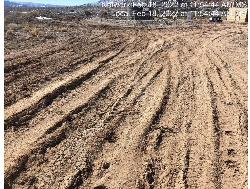
Photo #5991 Location lacks stabilization.
