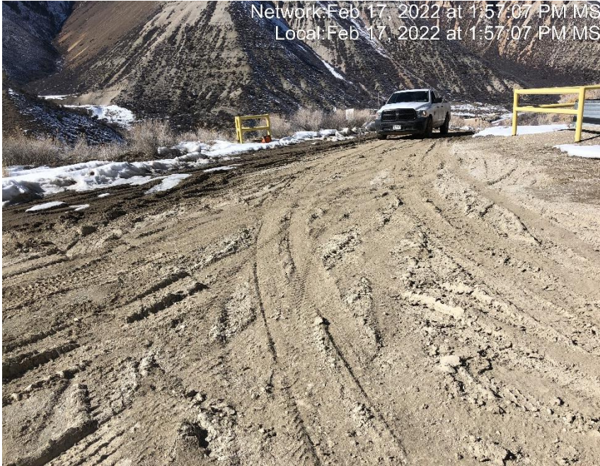
Photo #5987 Insufficient tracking BMP's at entrance to location.
