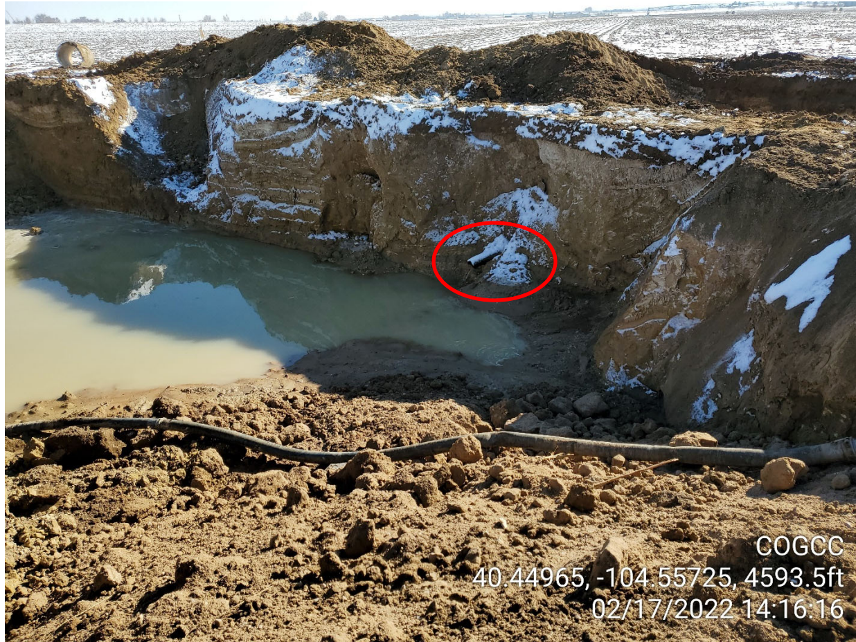
Photo 2: Looking at south wall of excavation. Field drain or other utility exposed in wall of excavation.
