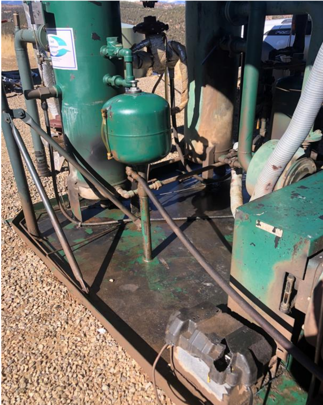
PHOTO 2: THE LEAK ON THE COMPRESSOR WAS REPAIRED. ALL FITTINGS ARE SECURLY FASTENED AND THE FLUID ACCUMULATION WAS REMOVED FROM THE CONTAINMENT. THE IMPACTED SOIL NEAR THE LIQUID RING COMPRESSOR WAS REMOVED AND PROPERLY DISPOSED IN ACCORDANCE WITH THE OGRIS OPERATING WASTE MANAGEMENT PLAN.
