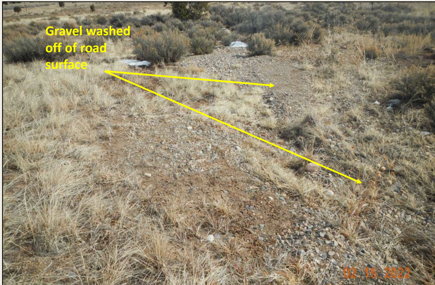
Photo 4. View of area down-slope from access road where gravel is washed off and deposited outside of the project area. Area is approximately 30ft long and 10ft wide.
