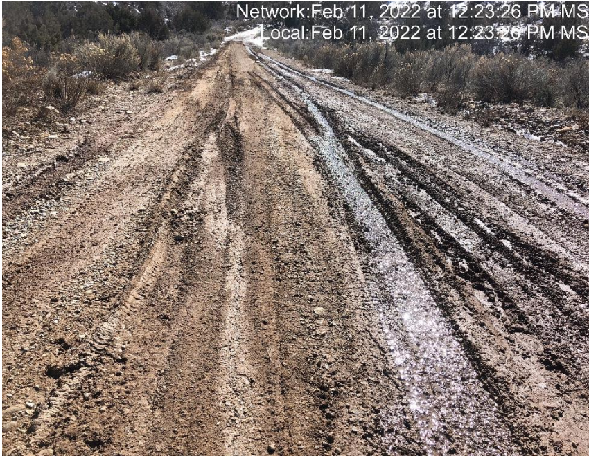
Photo #5941 Insufficient tracking BMP located at the entrance to location.
