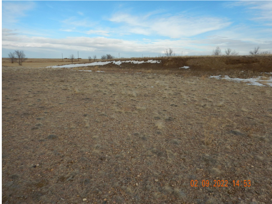
Photo 6. Photo taken from the eastern location, facing Northeast. Photo illustrates the topsoil stockpile. Topsoil stockpile was not properly stabilized. There was some erosion evident along the west-facing side.
