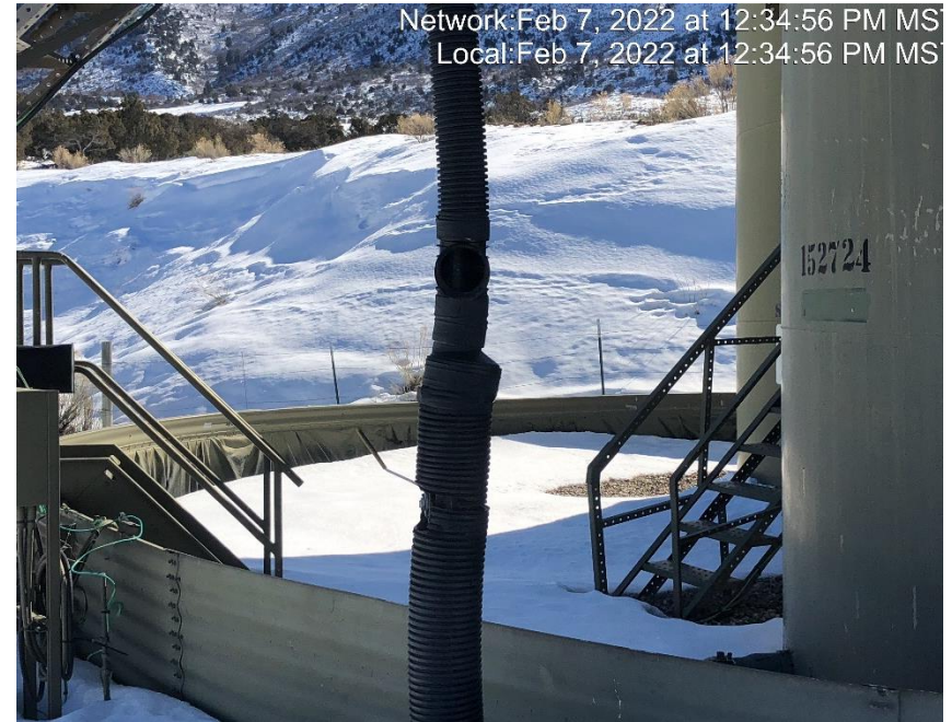
Photo #5886 Heating insulation open ended and not capped.
