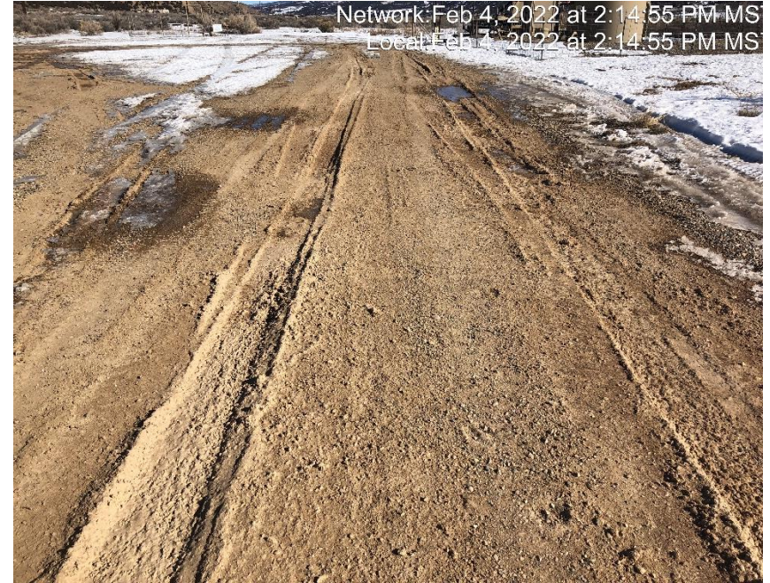
Photo #5881 Location lacks stabilization.
