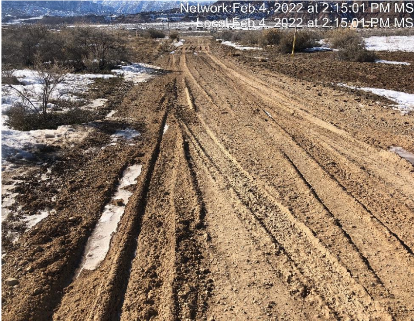
Photo #5882 Insufficient tracking BMP located at entrance to location.
