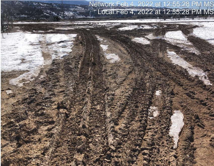
Photo #5872 Location lacks stabilization.
