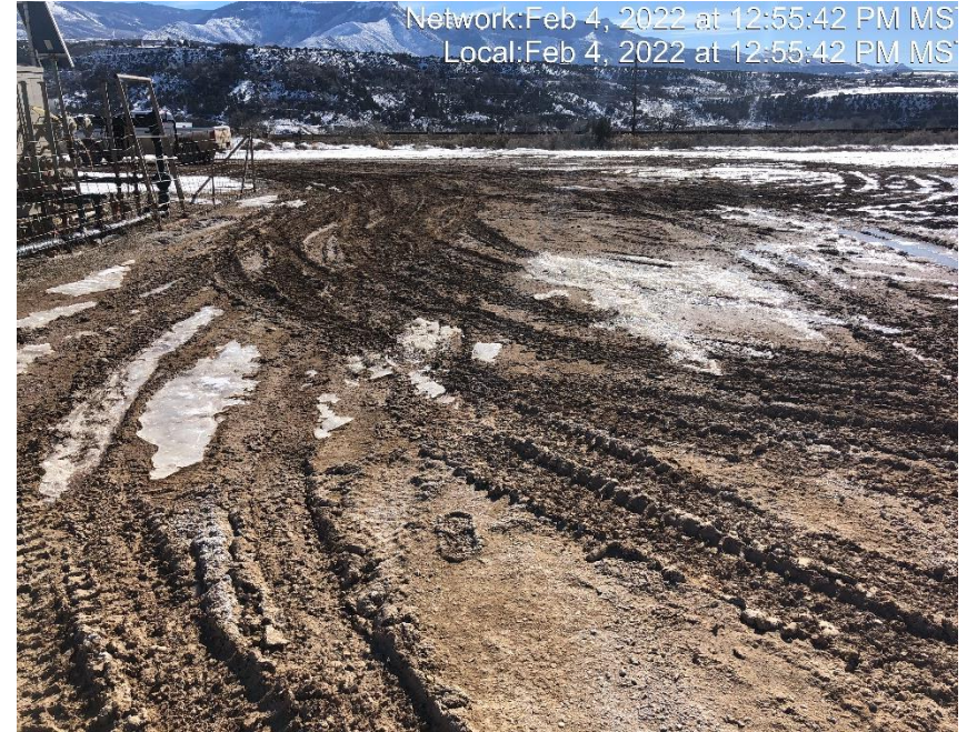
Photo #5873 Location lacks stabilization.
