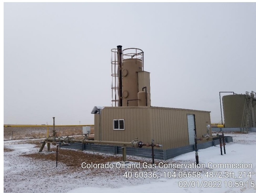
Photo 8 – Heater Treater and Gas Meters
