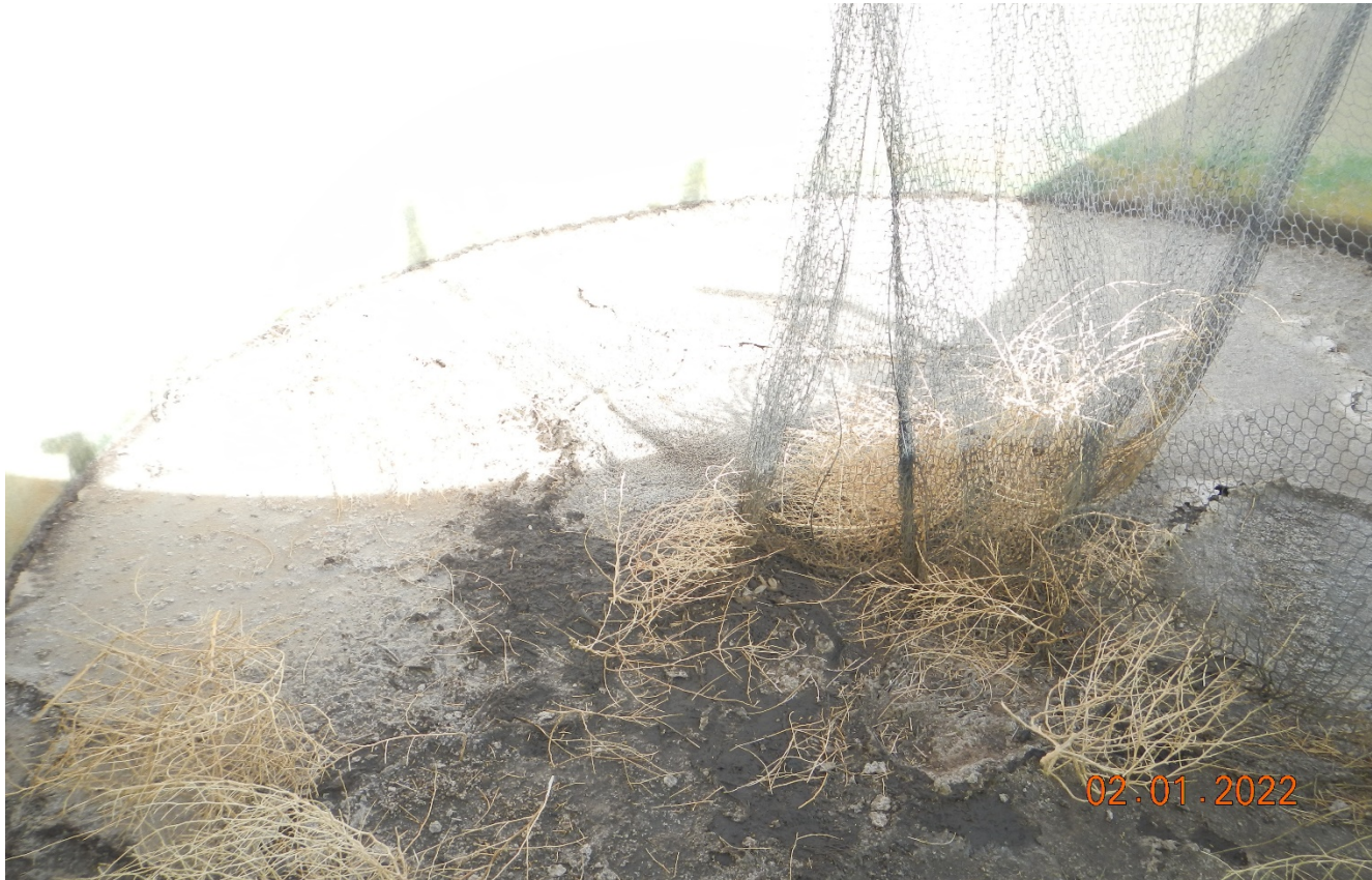
Photo 2. There is a solidified substance in the tank and the netting is not maintained.
