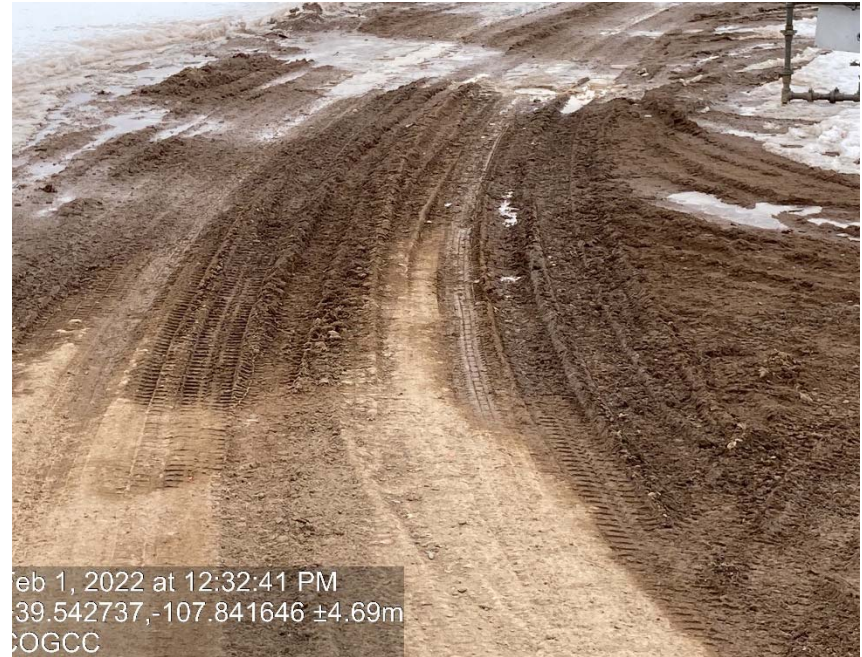
Lack of stabilization/compaction/degradation
