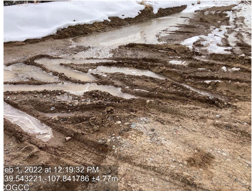
Lack of stabilization/compaction/degradation
