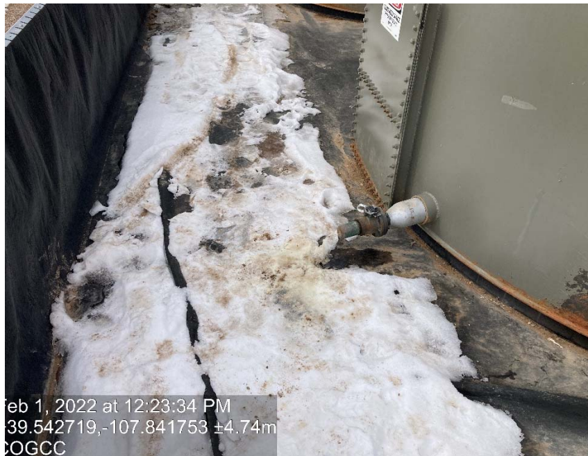
Staining under bull plugged load line
