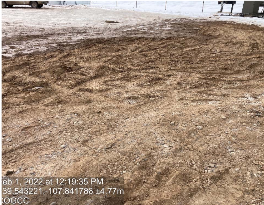
Lack of stabilization/compaction/degradation
