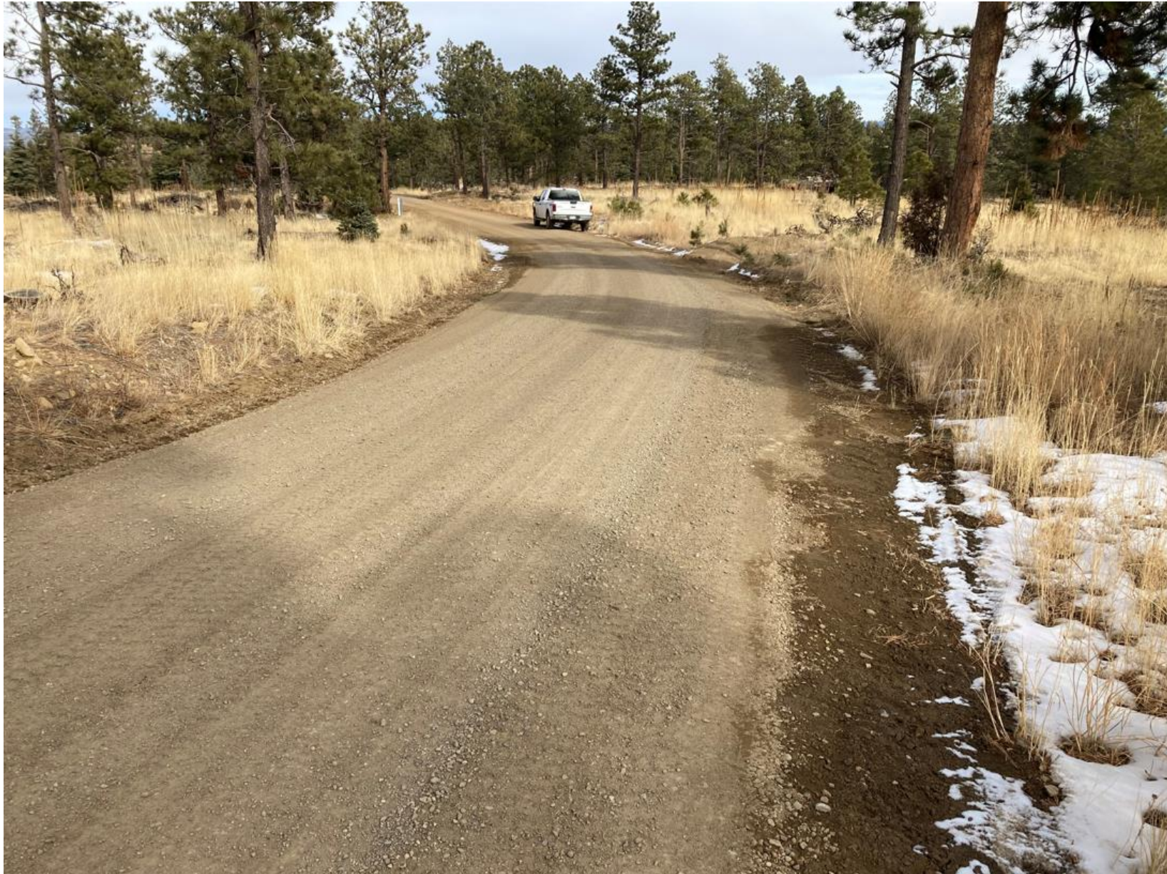
ADDITIONAL GRAVEL WAS INSTALLED TO THE ROADWAY SURFACE FOR STABILIZATION.
