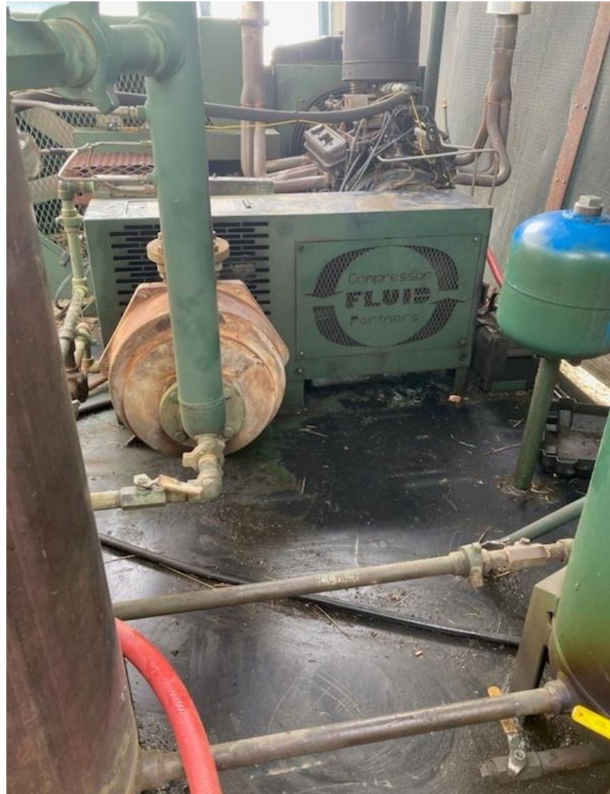
PHOTO 2: THE LEAK ON THE COMPRESSOR WAS REPAIRED. ALL FITTINGS ARE SECURLY FASTENED. THE FLUID ACCUMULATION WAS REMOVED FROM THE CONTAINMENT. COMPLETED 02/01/2022.
