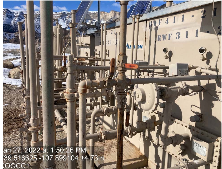
1 inch dump line leaking out of the top past valve
