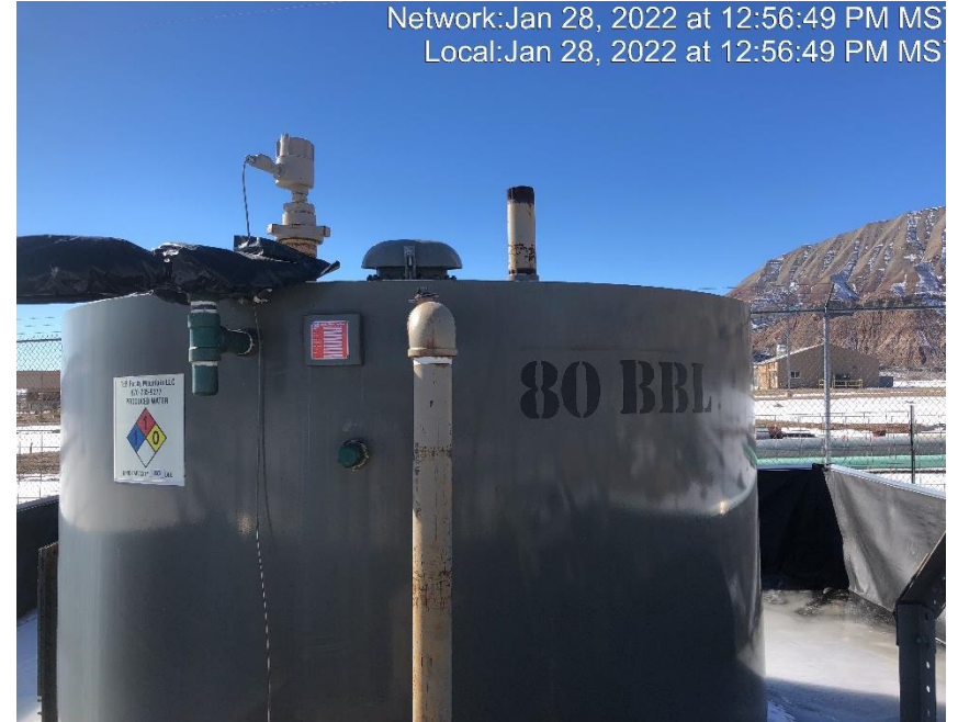
Photo #5819 Vent pipe on tank open ended.
