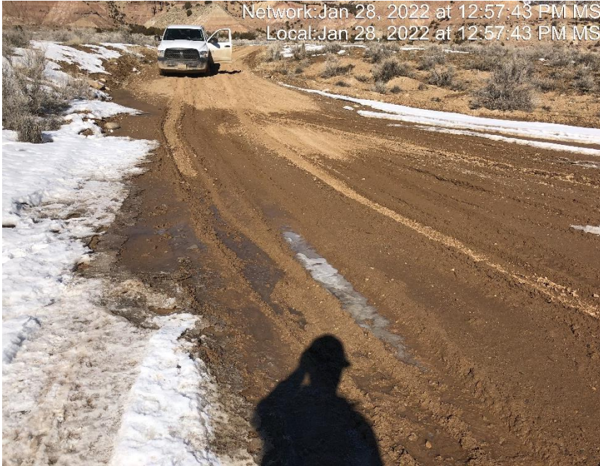
Photo #5822 Insufficient tracking BMP located at the entrance to location.
