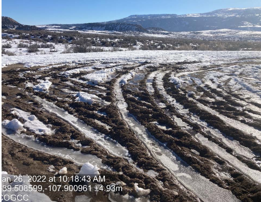
Lack of stabilization/compaction
