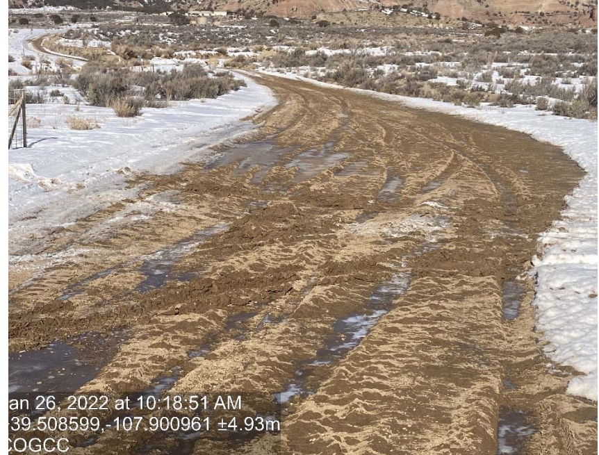
Lack of stabilization/compaction
