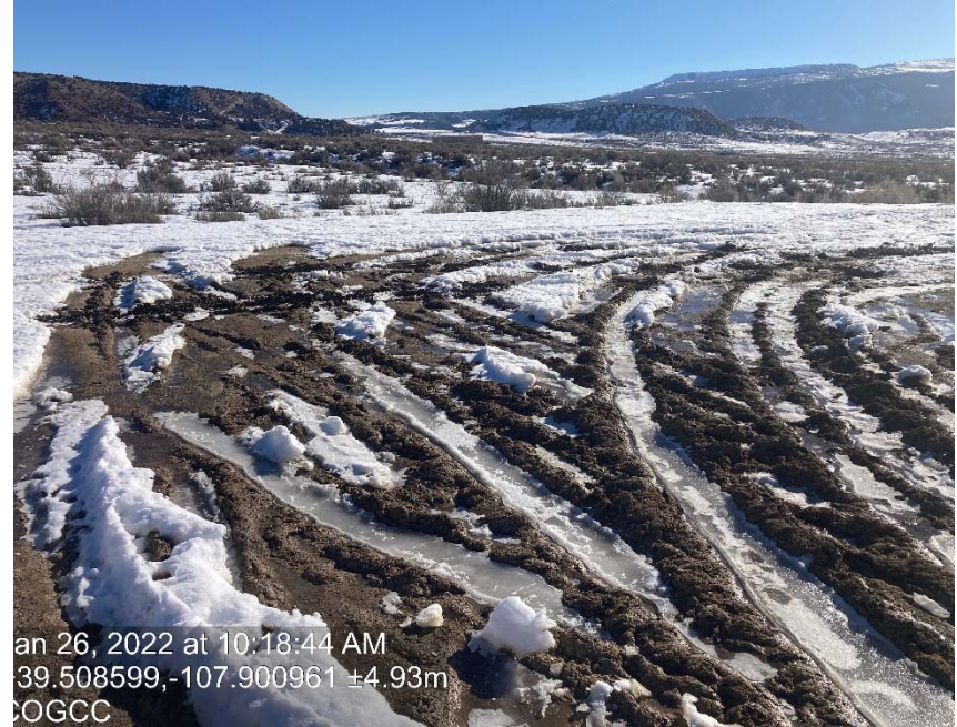
Lack of stabilization/compaction
