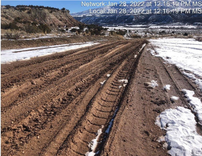
Photo #5817 Insufficient tracking BMP at entrance to location.
