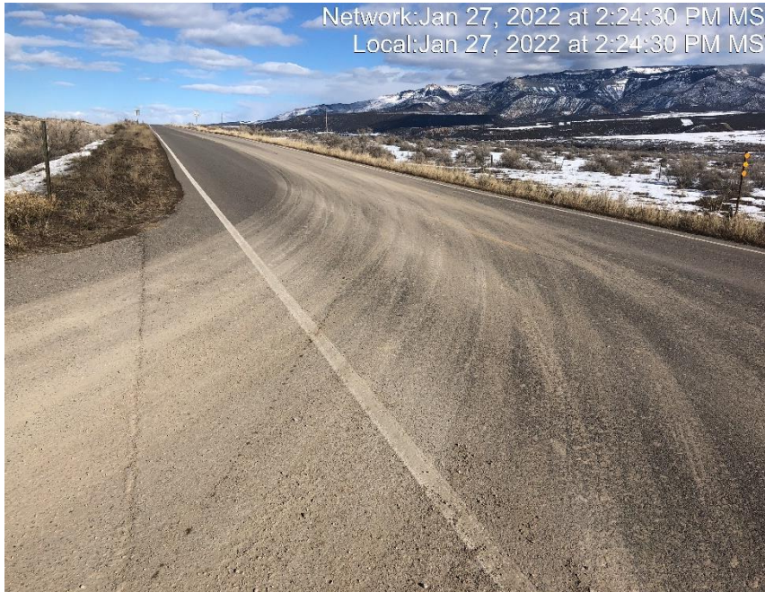
Photo #5811 Tracking occurring from access road on to highway 6.
