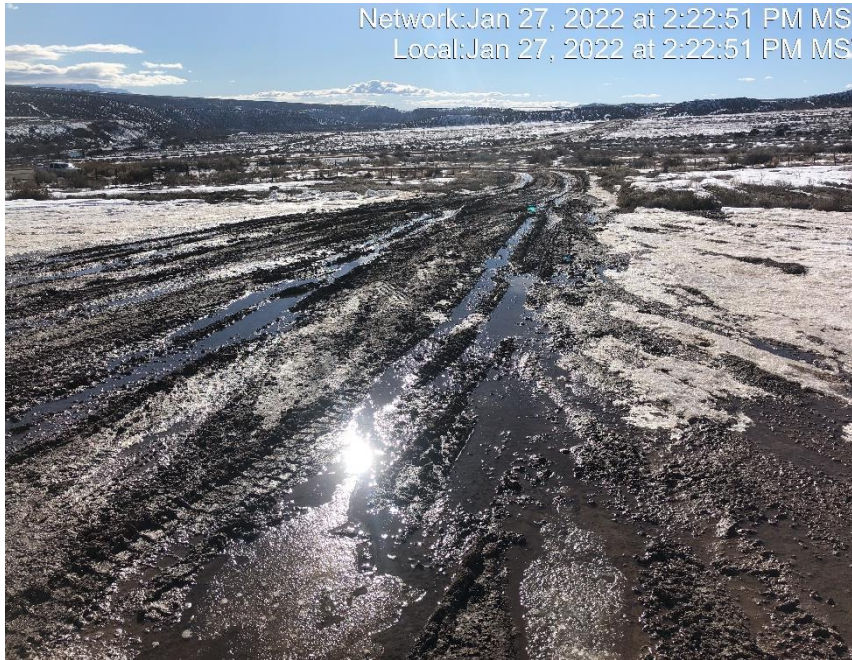
Photo #5807 Access road lacks stabilization.
