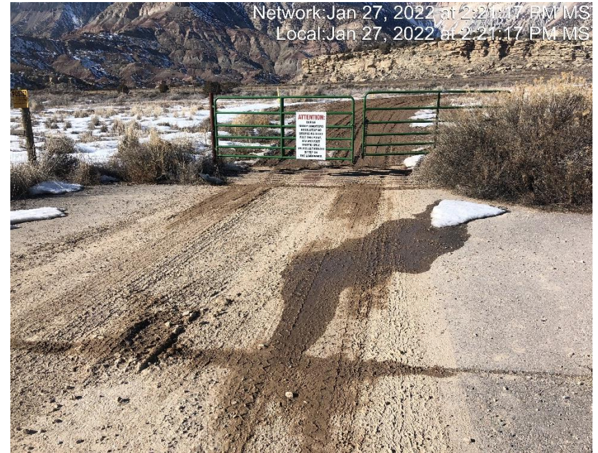
Photo #5804 Insufficient tracking BMP located at entrance to location.
