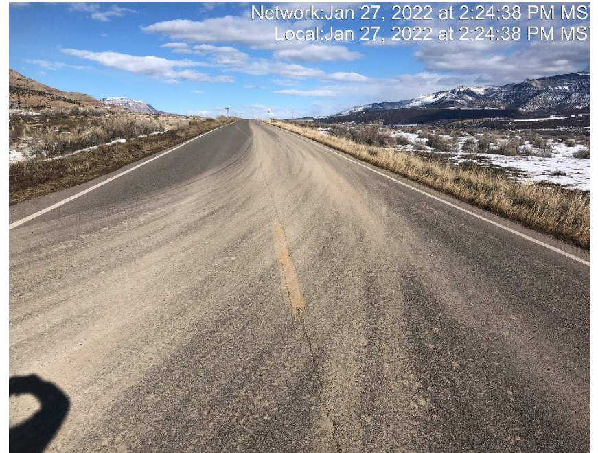
Photo #5812 Tracking occurring from access road for approximately 100 yards.
