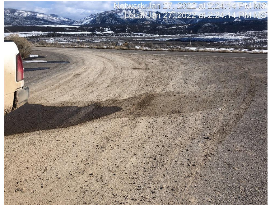
Photo #5810 Tracking occurring on to highway 6.
