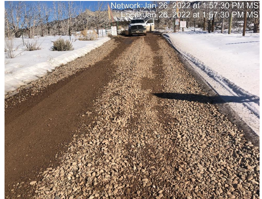
Photo #5797 Insufficient tracking BMP.
