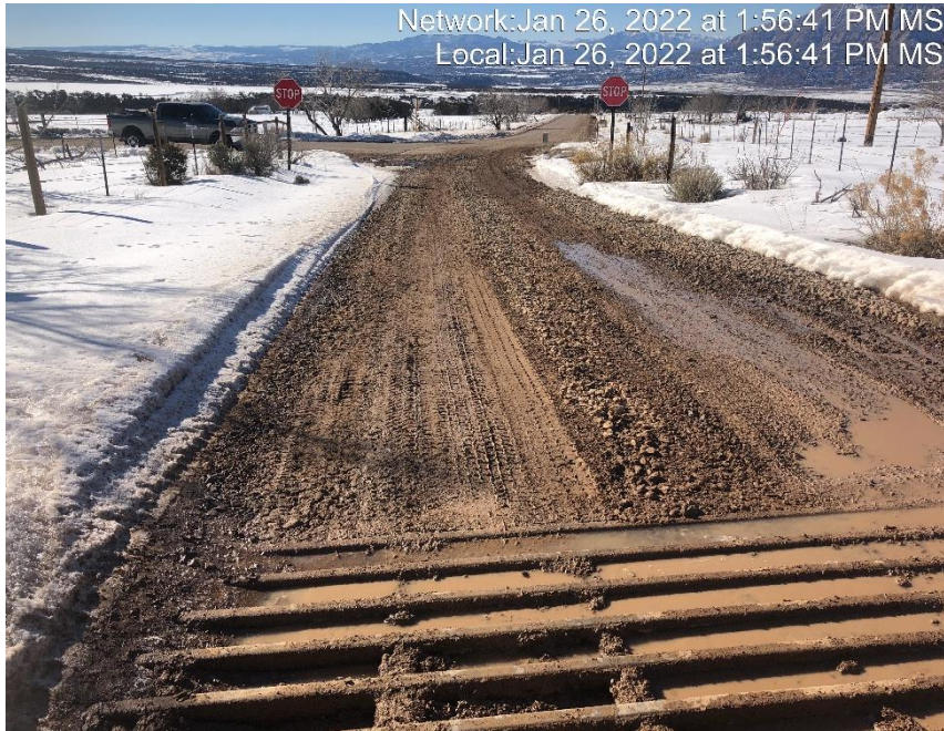
Photo #5793 Insufficient tracking controls.
