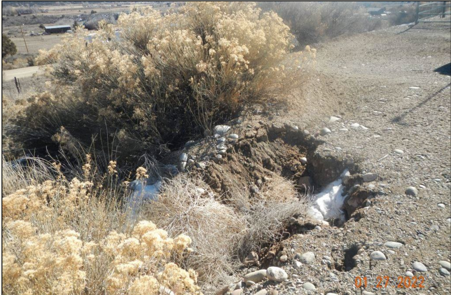
Photo 4. View of erosional tunneling occurring where concentrated stormwater flows off of the northeastern corner of the well pad around and below a cobble BMP that is not functioning properly.
