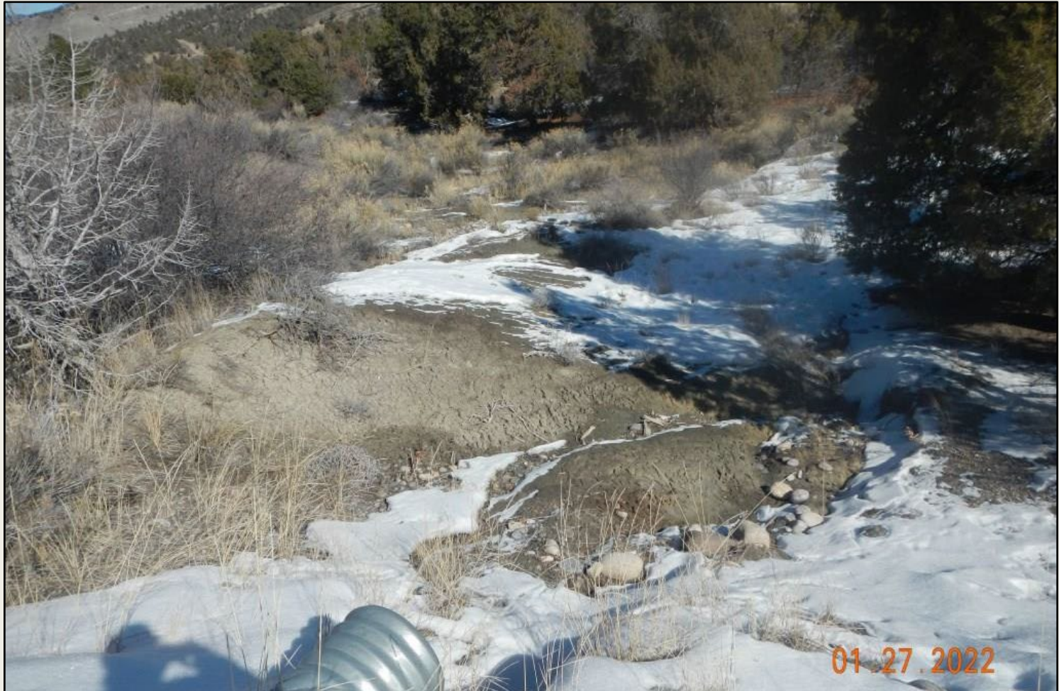
Photo 7. View of area downslope from culvert outlet near well pad entrance where multiple erosional channels are eroding the slope without adequate stabilization.
