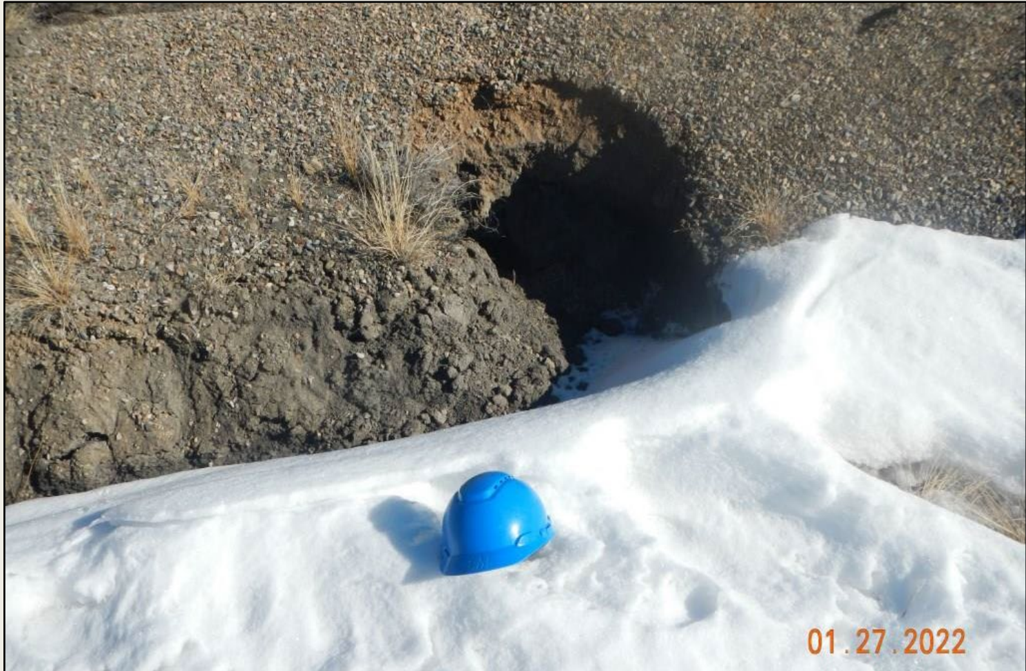
Photo 4. View of erosional tunneling within the northern fill slope where concentrated stormwater tunnels through well pad berms. Hard hat in place for scale.
