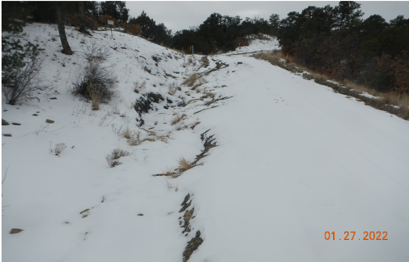
Photo 3. The is areas of erosion along the road side traveling to the location.
