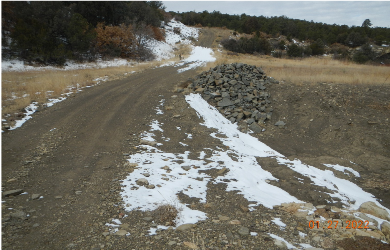
Photo 2. Facing northwest toward the access road. There is a pile of rock rip/rap which appears to have been placed here for bank stabilization and stormwater repairs.
